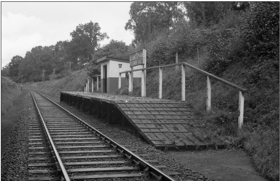
Below: Llanstephen Radnor Halt looking north on 4 September 1962; the Halt dates from 1933
