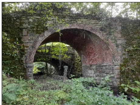
Rail and road bridge at SS 799905;
