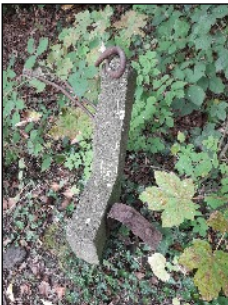
Incline overbridge at SS 752951
