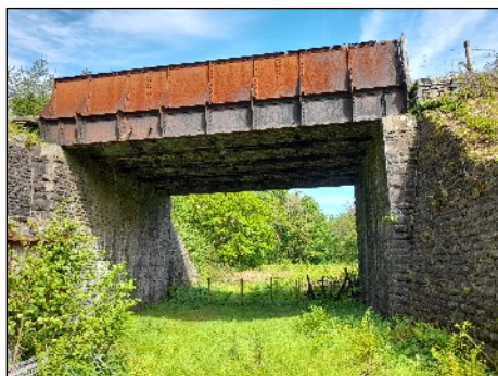
bridge at SS 958868
