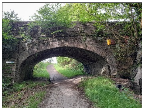
bridge at SS 975875
